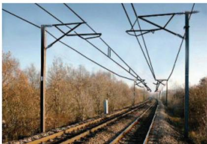
Overhead line equipment (OLE) provides trains with 25,000 volts AC. You must treat the OLE as being live at all times. Cables attached to these structure must be considered to be live as well.
