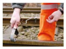
When setting out detonator protection the detonators must be attached to the running rail furthest from the conductor rail
