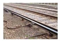
The conductor rail and any of its connections must be treated as live and dangerous at all times.
